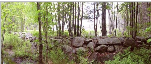
Stone work along the dam at Converse Meadow, at the old mill site.
